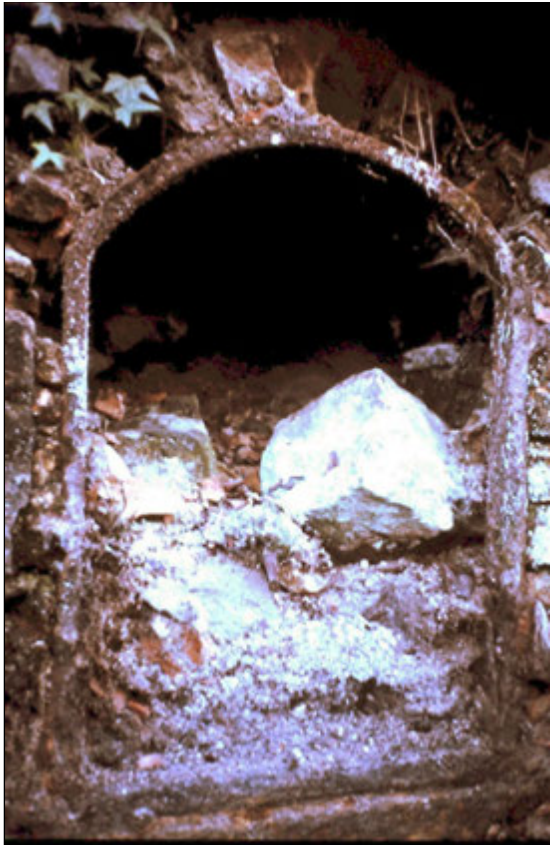
Arsenic Works furnace door (photograph by John Hayman, November 1985)
