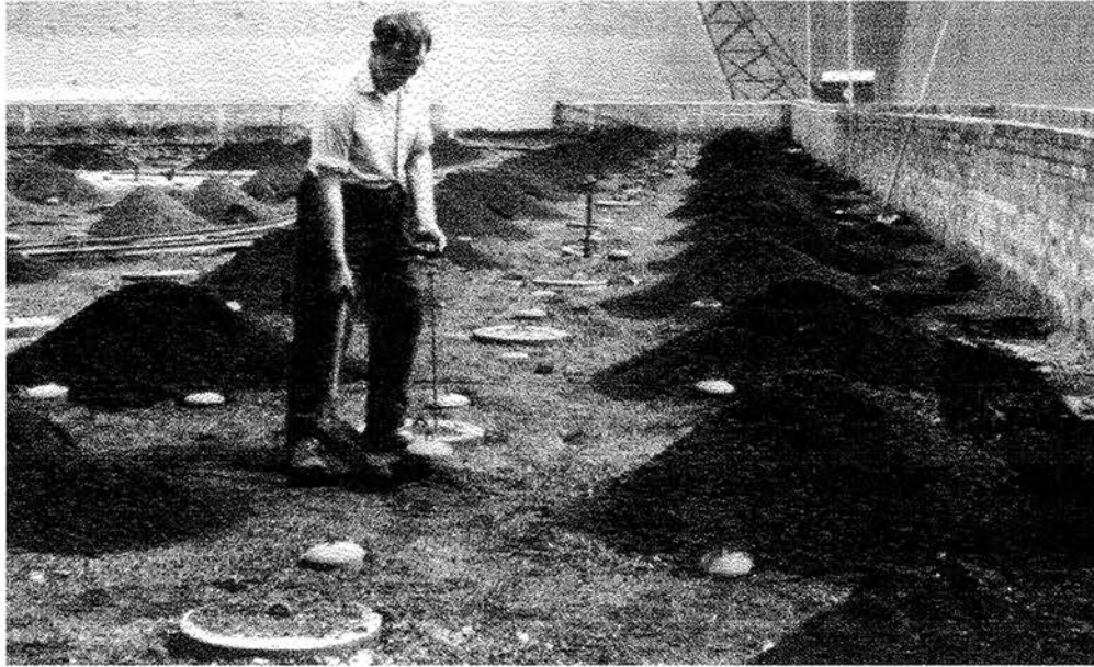
Fig.31. Roof of continuous kiln illustrating coal, spy holes and dampers as remembered by Roberts
